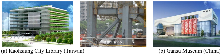
Figure 3 Application of sandwiched BRBs in Taiwan and China.
