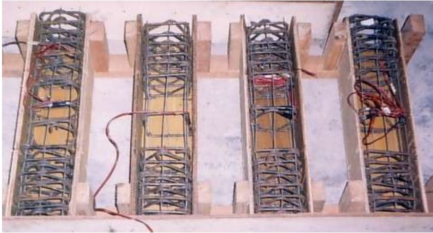
Figure 3 Typical reinforcement cages for confined concrete.
