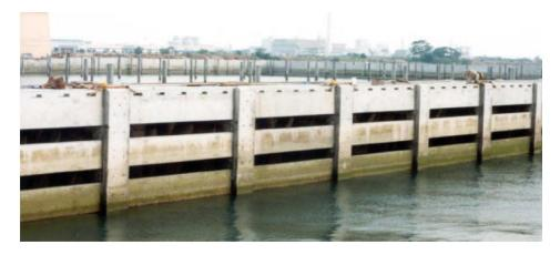
**Figure 2** Example of the application of perforated breakwater (Raffles Marina Wharf/breakwater in Singapore).
